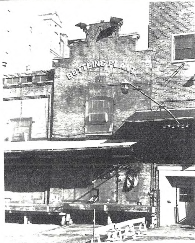
Bottling plant (see if you can find this building in the 1905 scene)
